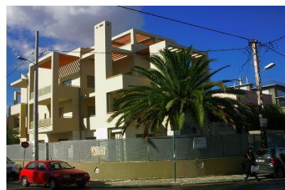
Cooling & Heating with DAIKIN VRF System in luxury building (Filothei)
